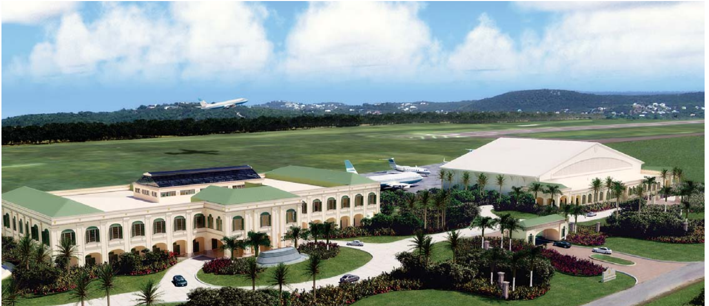
Ground was recently broken on the Stanford Global Headquarters in St. Croix, United States Virgin Islands. The 37-acre campus is expected to be completed in late 2009.
